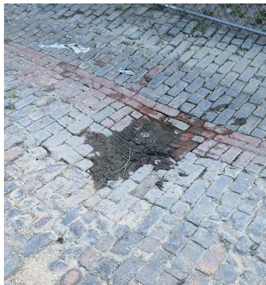
Picture 15: Sinkhole in Alley.
