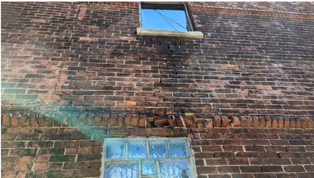
Picture 8: Crack Between Windows in West Wall
