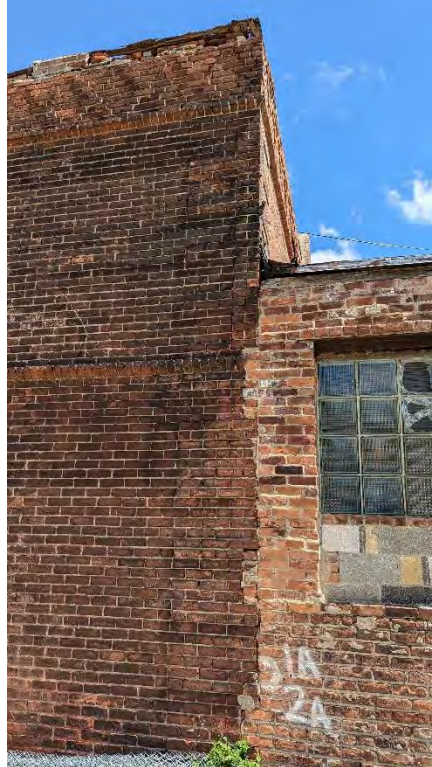
Picture 11: Crack Along Intersection of Walls at Southwest Corner.
