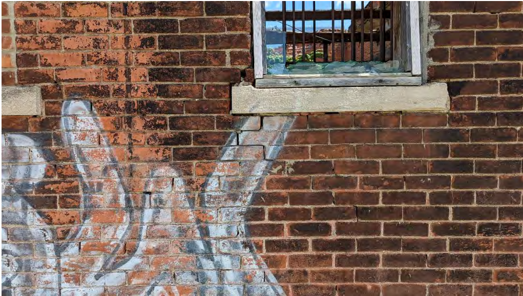
Picture 7: Crack Below Window in West Wall
