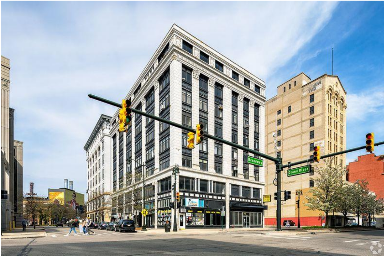
206 E. Grand River (Merchants Building) 6
