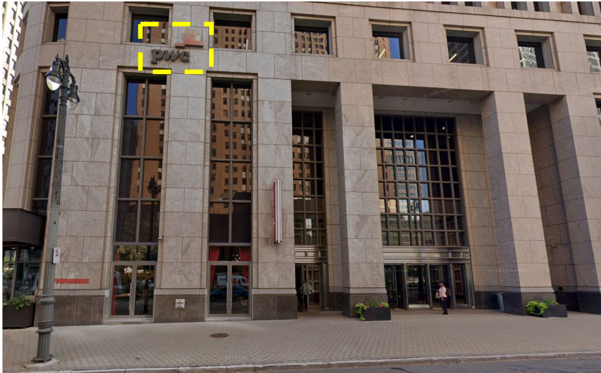
Existing wall sign to be replaced
