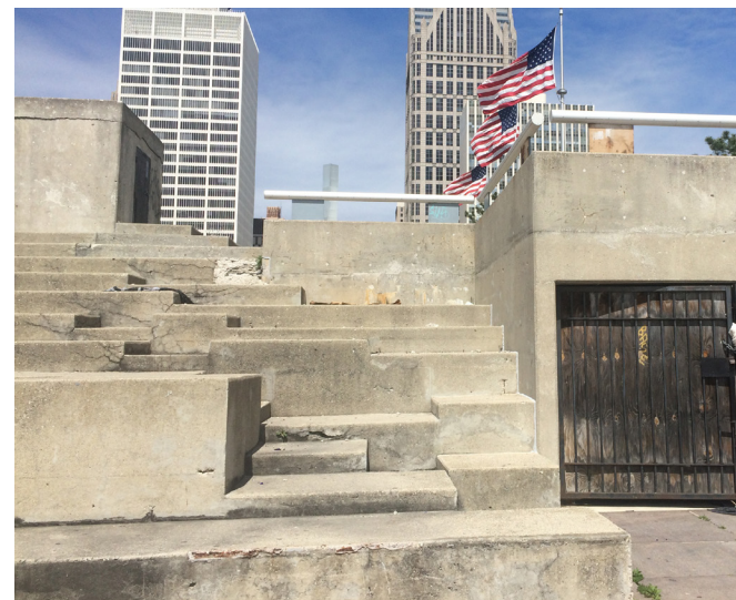
The mass concrete structure (Pyramid) is in poor condition and poses a safety hazard
