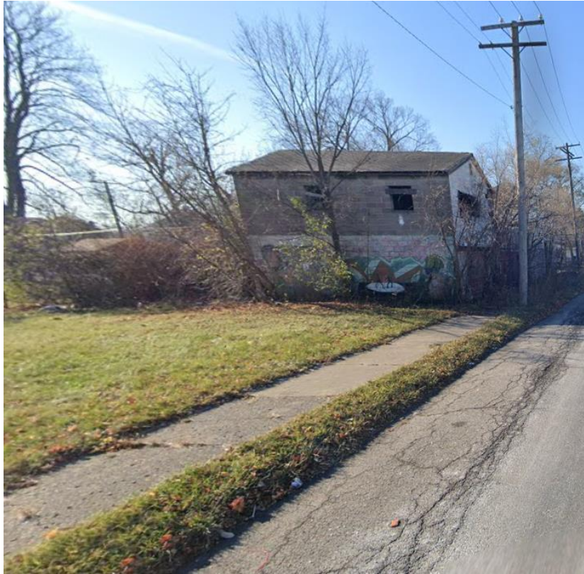
Existing site as viewed from the corner of 16 th Street and McGraw (looking southeast).
