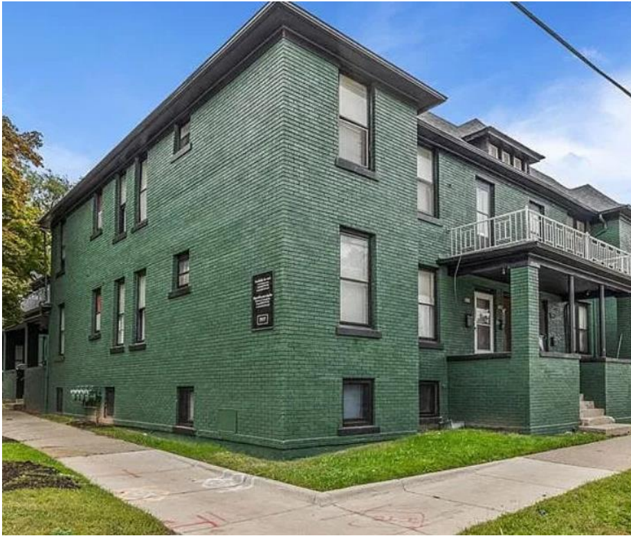
Existing building as viewed from the corner of Campbell and Toledo (looking southwest).
