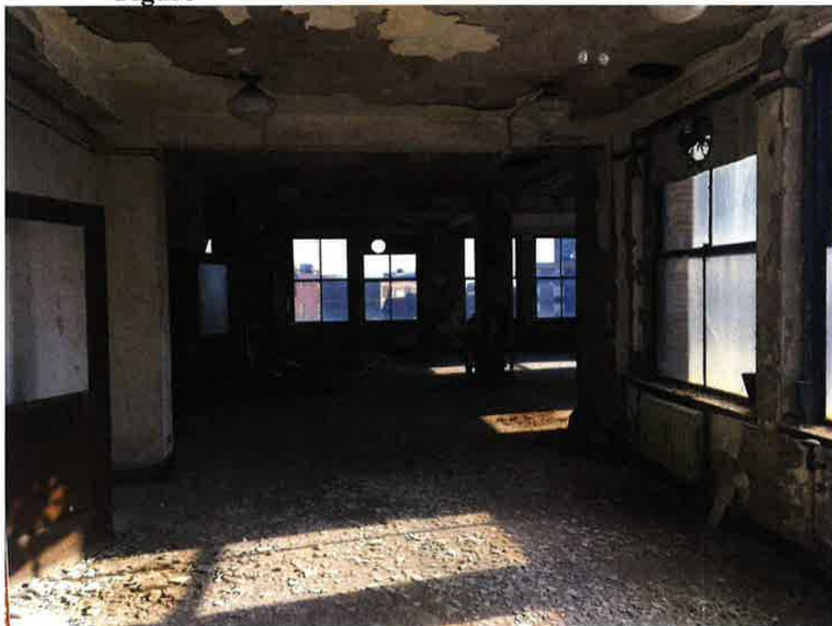
Figure B.9: Pre-Rehabilitation Interior Conditions
