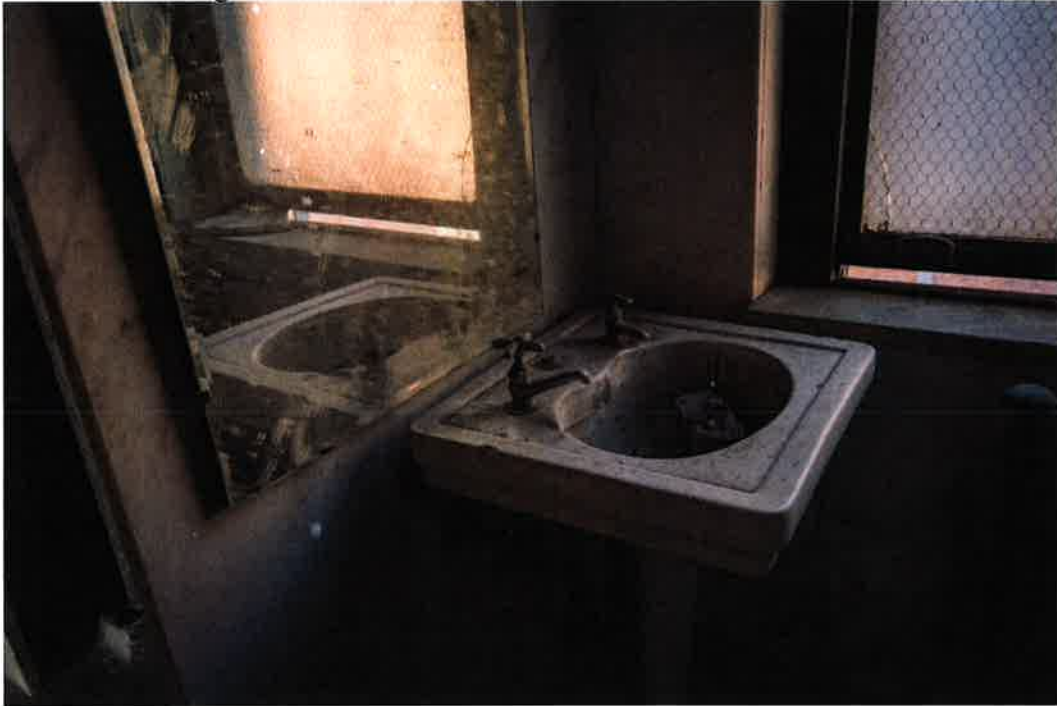
Figure B.6: Pre-Rehabilitation Interior Conditions
