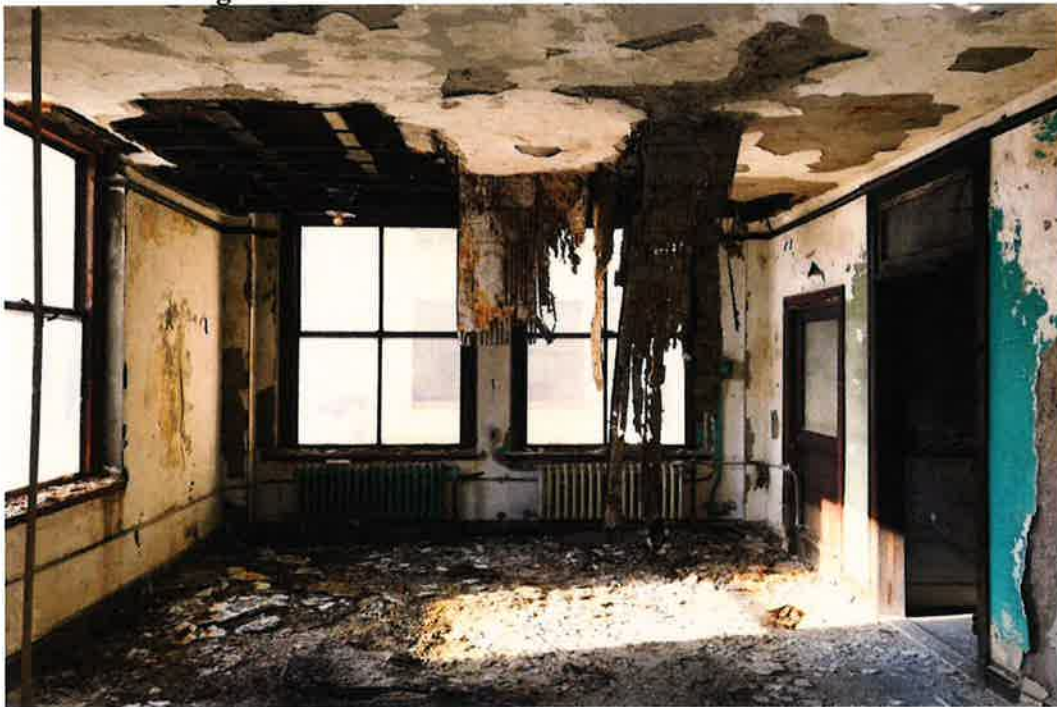
Figure B.3: Pre-Rehabilitation Interior Conditions
