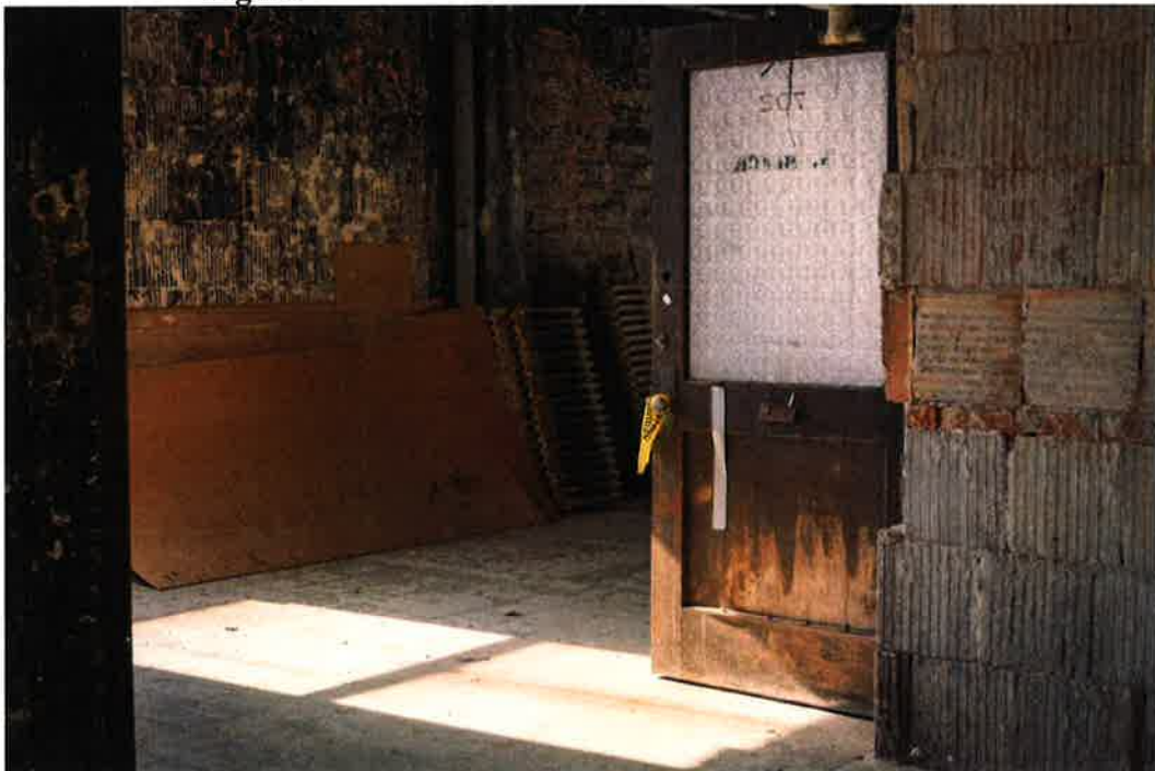
Figure B.7: Pre-Rehabilitation Interior Conditions
