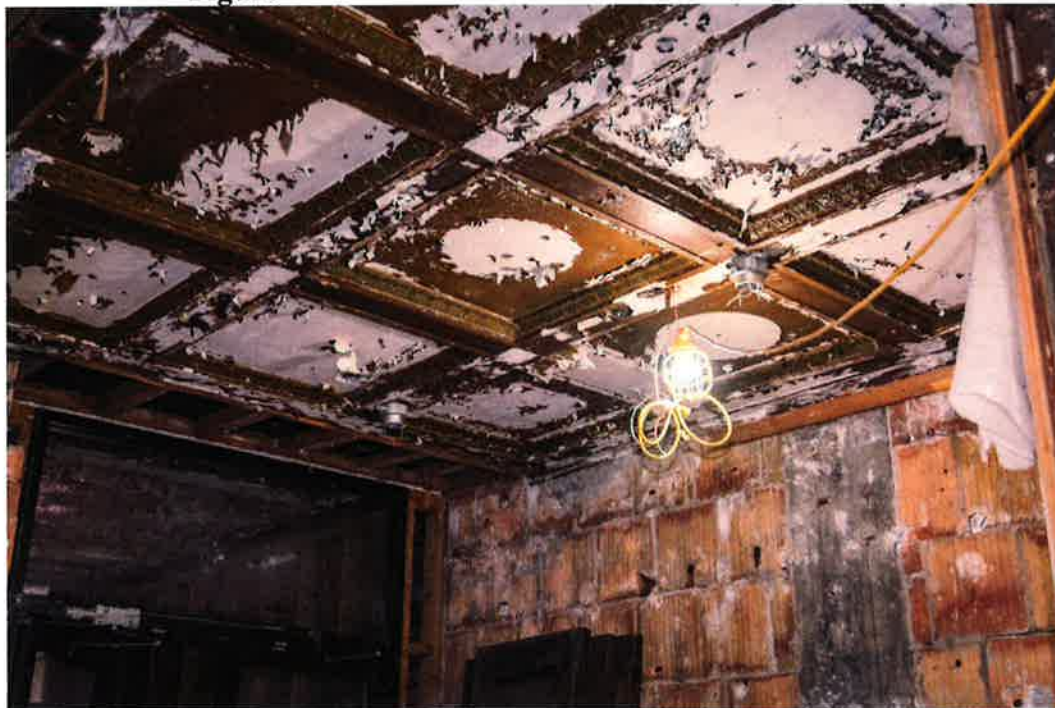
Figure B.5: Pre-Rehabilitation Interior Conditions
