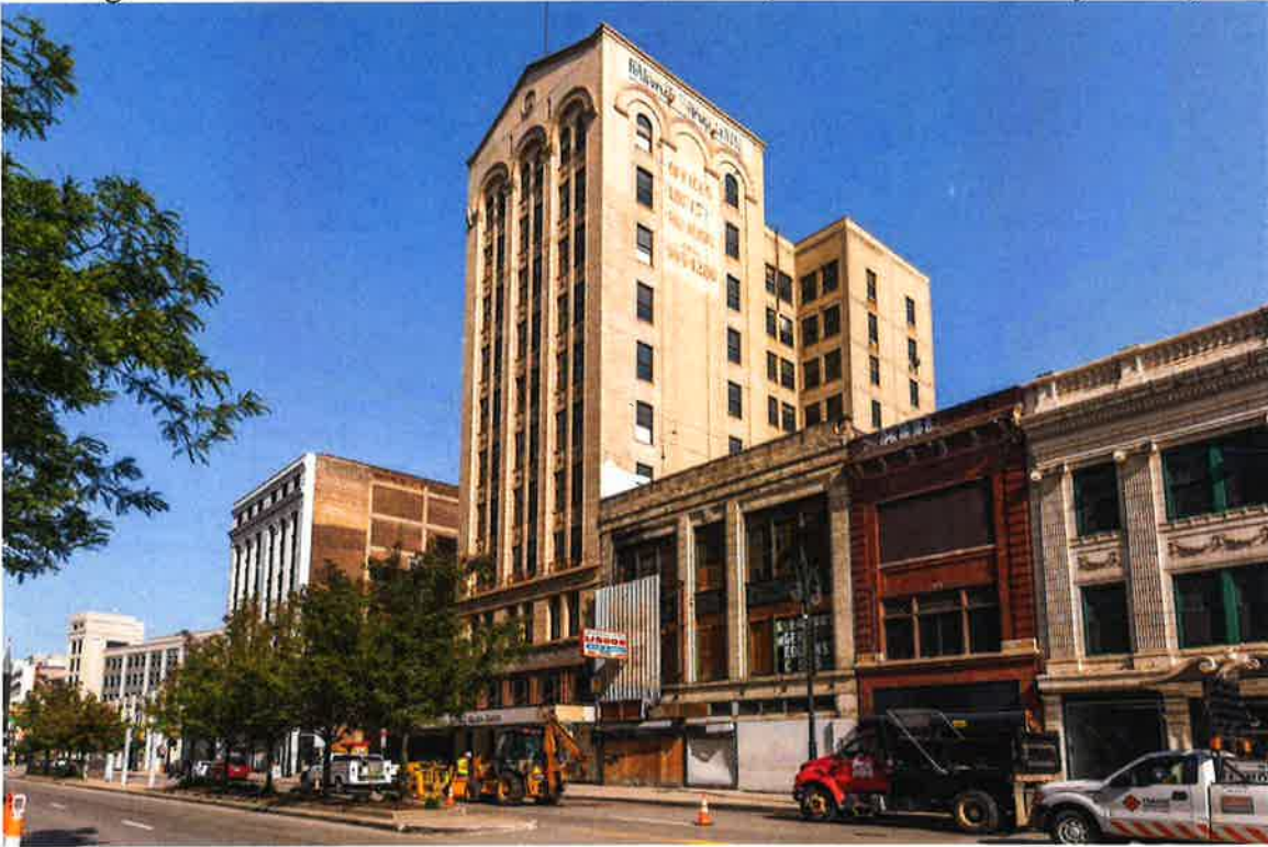
Figure B.2: Pre-Rehabilitation Exterior View (view from Broadway Street)
