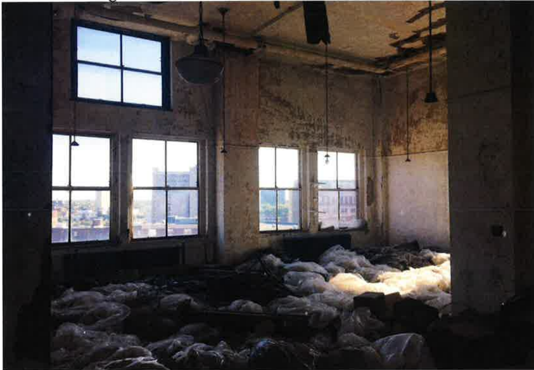
Figure B.4: Pre-Rehabilitation Interior Conditions
