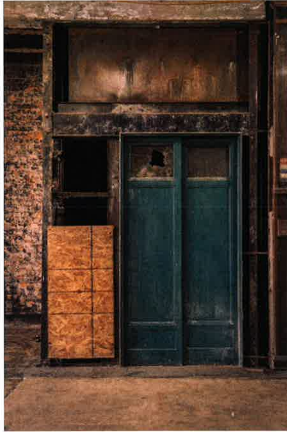
Figure B.10: Pre-Rehabilitation Interior Conditions
