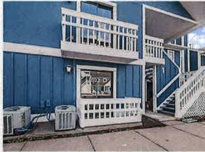
Exterior Painting & Balconies
