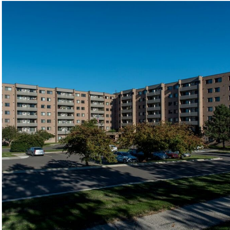
Cranbrook Tower Ann Arbor, Michigan
