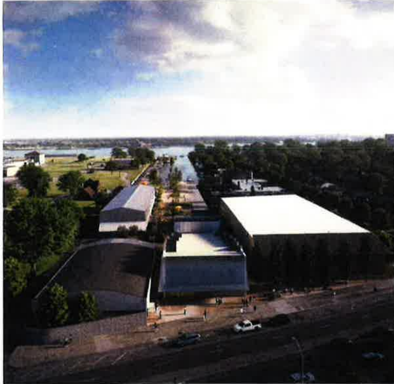
Aerial street view of buildings fronting E. Jefferson Avenue
