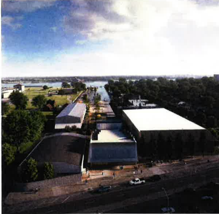
Aerial street view of buildings fronting E. Jefferson Avenue
