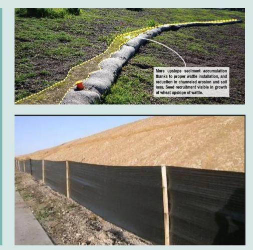
Filter strip pretreatment Geotextile filter fabric Soakage
