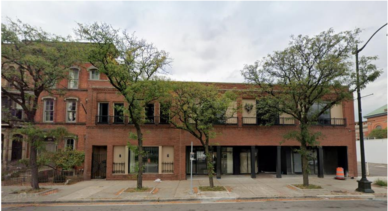
Front façade of the building facing Jefferson circa October 2023
