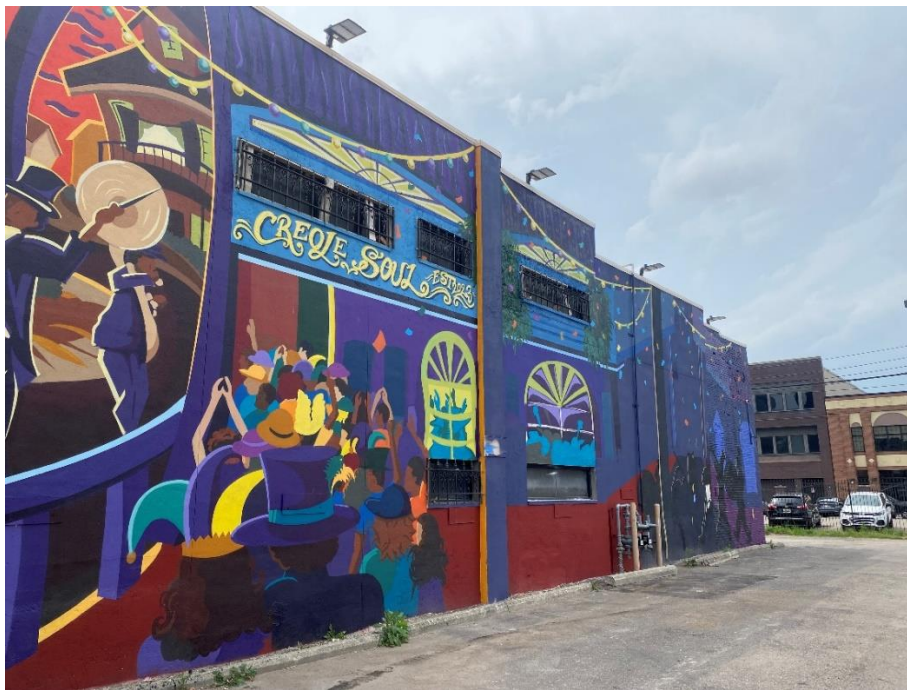
Mural painted on the east façade of the building but not included in the permit application
