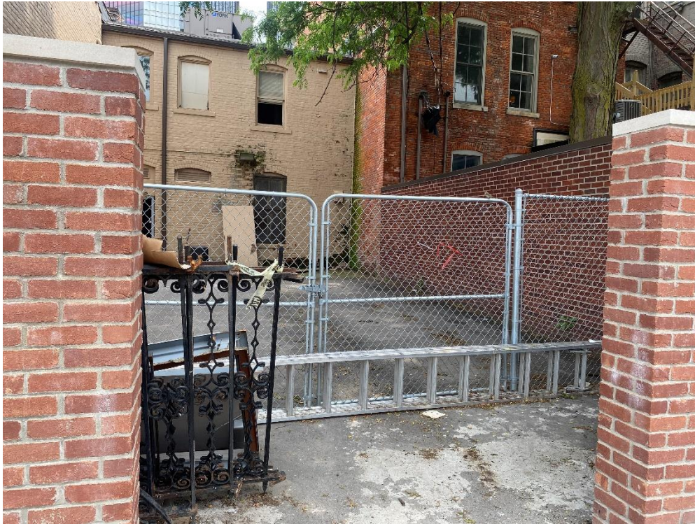
Newly constructed brick walls at the rear of the building
