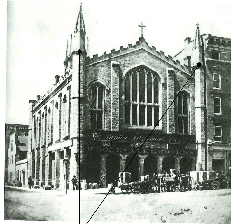
RECONSTRUCT NEW PINNACLES ON EXISTING TURRETS AT EACH OF 4 CORNERS OF THE CHURCH
